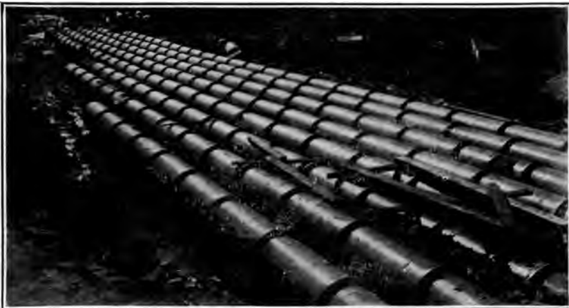
FIG. 2. — Pipe-line of New Croton Aqueduct. (8 lines of 48-inch cast iron pipes.)
